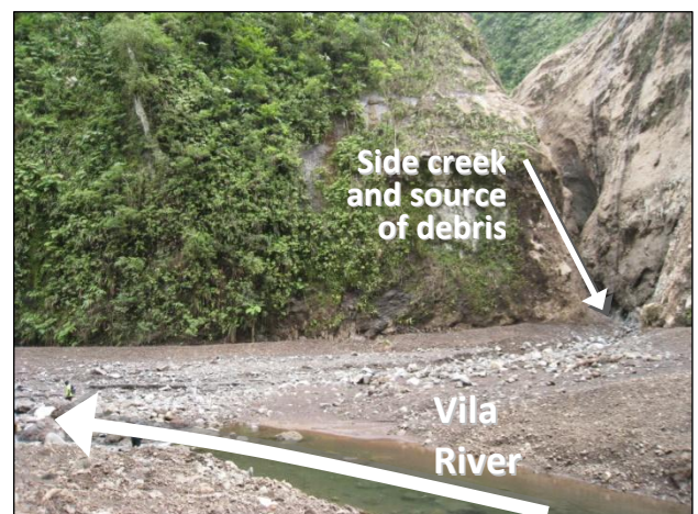
Side creek (far right) brings silt from Mt Rano landslide and blocks Vila River. Lower end of new 400m pool in foreground. Earlier in the year this section of river was free-flowing. If you want to see the new pool, you had better be quick! We expect summer rains to remove the blockage in the coming months. (continued over)
